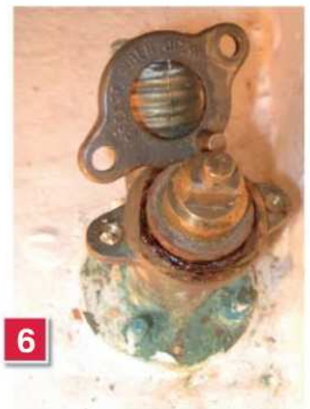
6 With both bolts removed, I lifted the keep plate from the body. At this stage it may in some cases be possible to lift the cylinder out from above, but...
